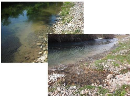
Figure 1. Leakage and fine particles erosion at the earth dam toe (Bourg-lès-Valence, 2007).
