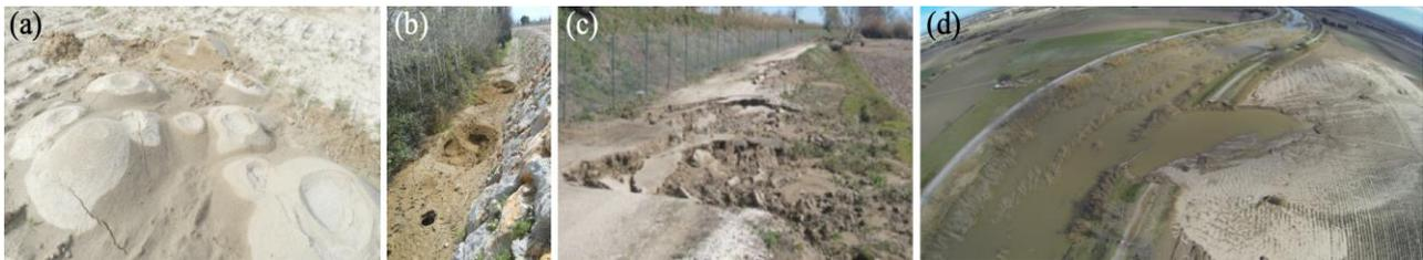
Figure 1. Examples of erosion signatures observed in 2012, 2013, 2014 at the vicinity of dikes at the Agly river during floods: sand-boils (a), sinkholes (b,c), gravitational collapses (d) (Photos INRAe).
