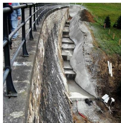
Figure 5. The reconstruction of the abutments after the flood in 2010.
