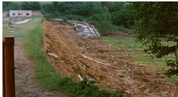
Figure 3. Downstream slope after the flood in 1996.
