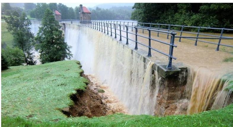
Figure 4. Overtopping of the dam Mlýnice during the flood in 2010.
