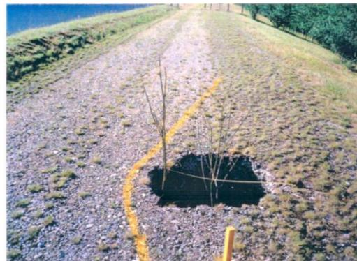
Figure 2. Sinkhole development on the dam crest (Brégner-Cordon, 1991).
